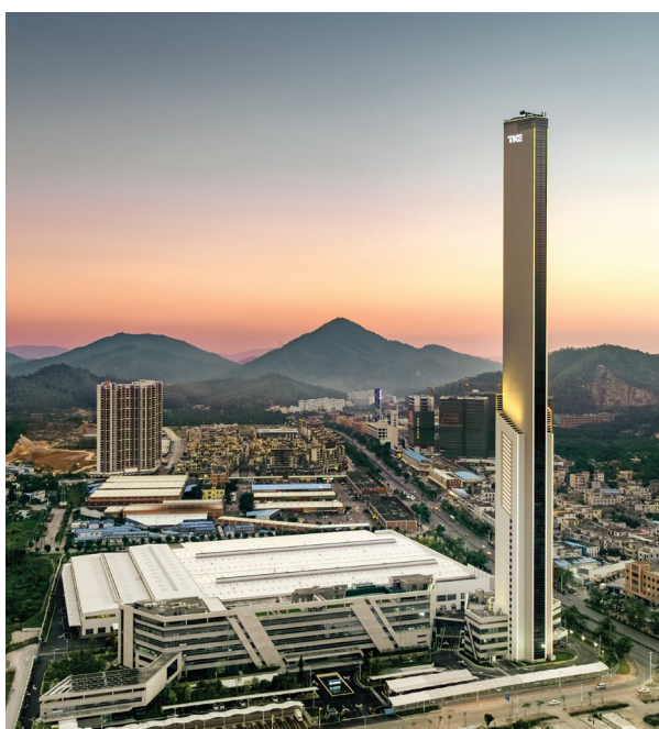
Torre de Testes - TK Elevator Zhongshan, China
